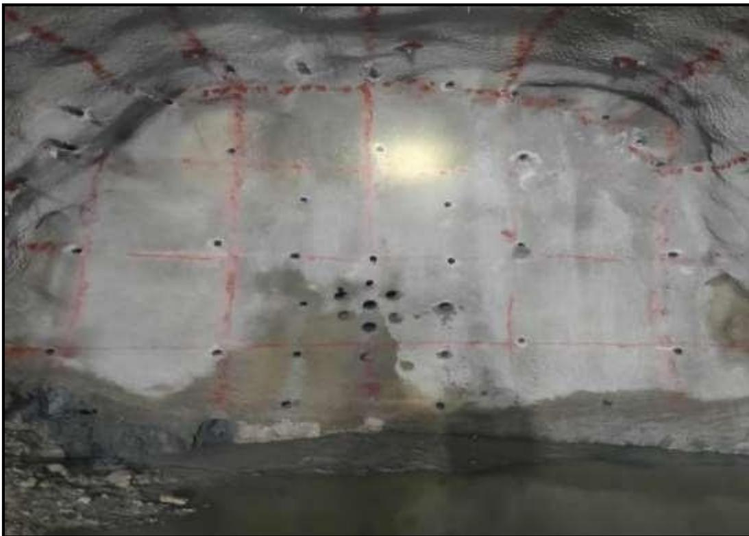
**Figura 41 — Frente perforado 4.50 m x 4.20 m**
