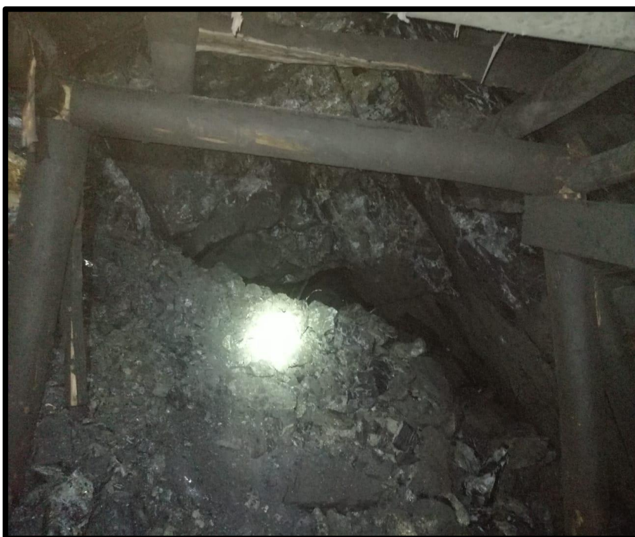
Figura 39 — Post-limpieza GL 599 Nv 8
