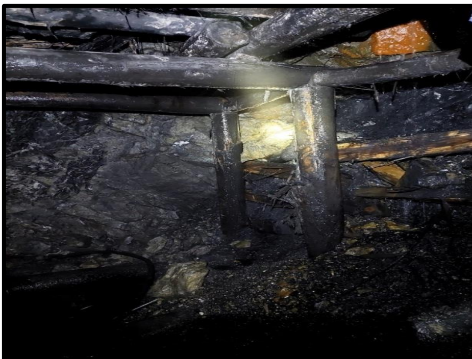
Figura 38 — Post-voladura GL 599 Nv 8
