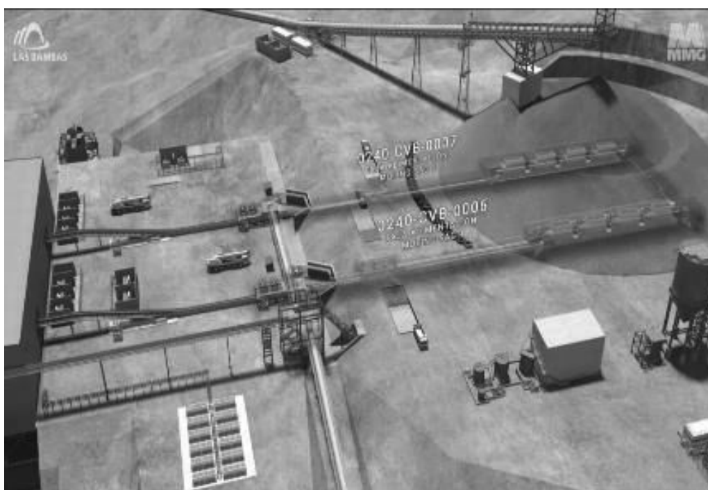
Figura 126. Area de Stock Pile
